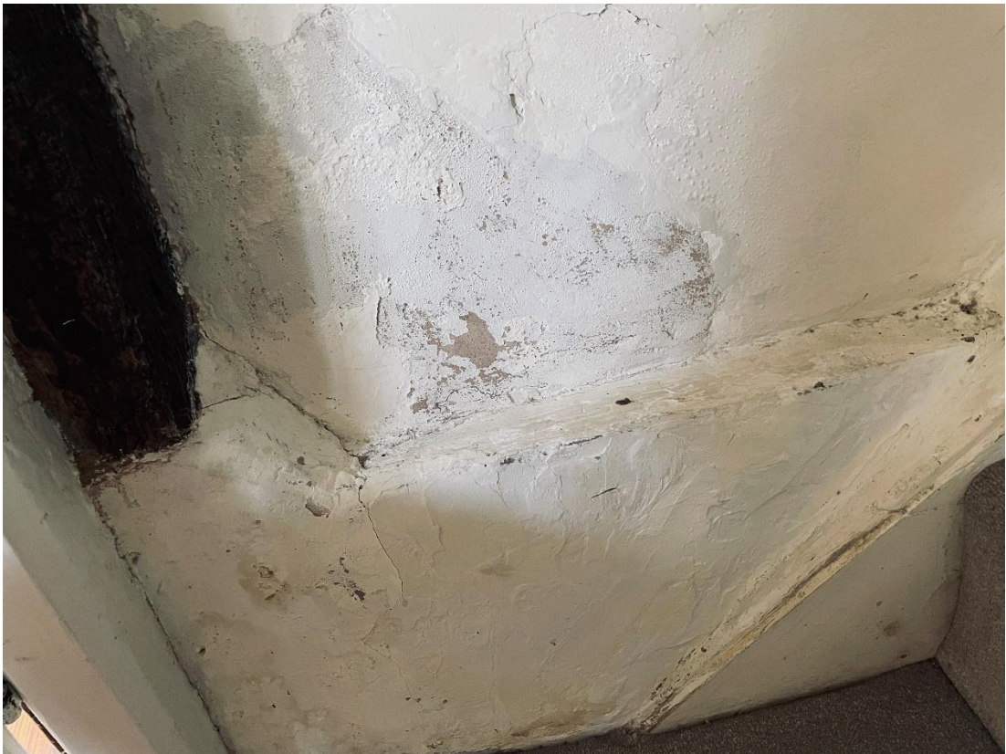
Dampness to the base of the stairs.
