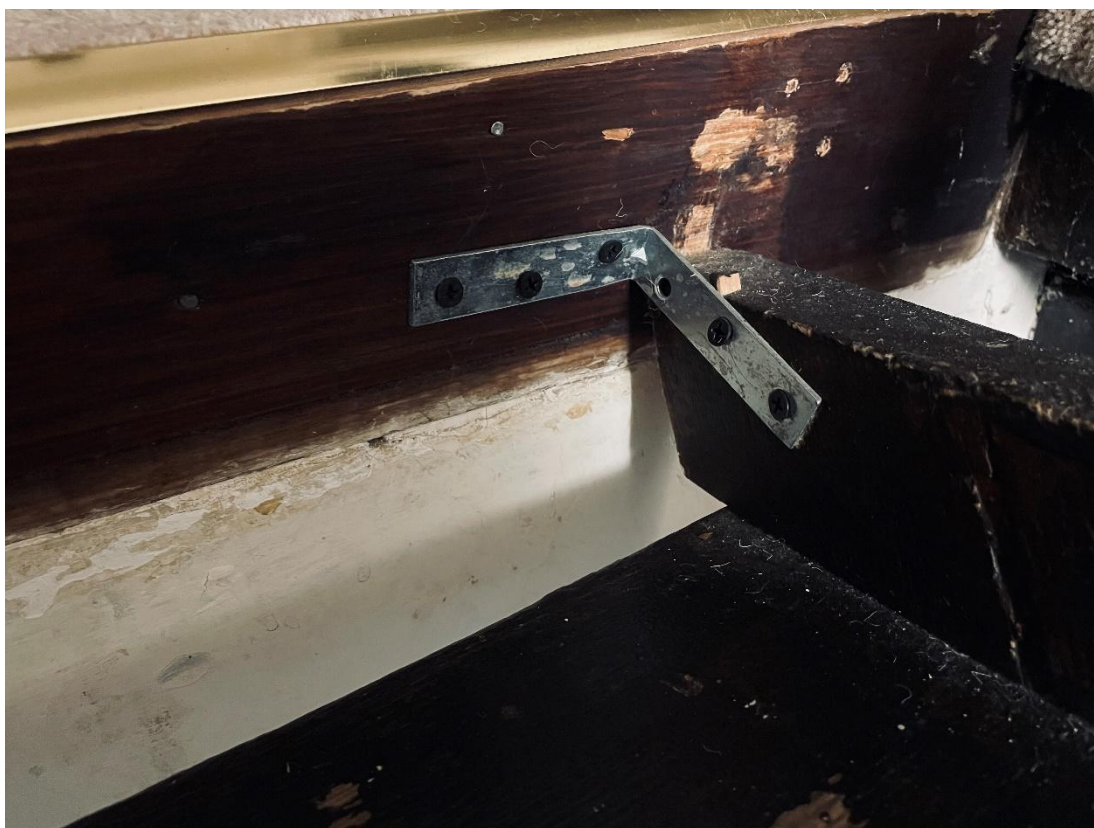
Inadequately supported ship's ladder.
