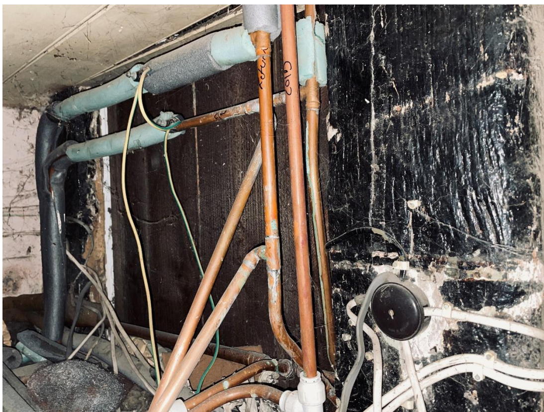
Uninsulated pipework in the loft over the entrance hallway.
