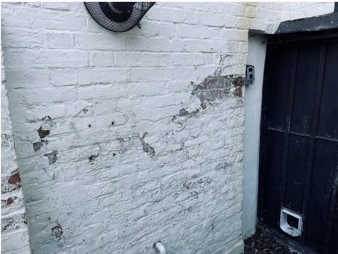
Peeling paint to the right-hand elevation of the front entrance hallway.
