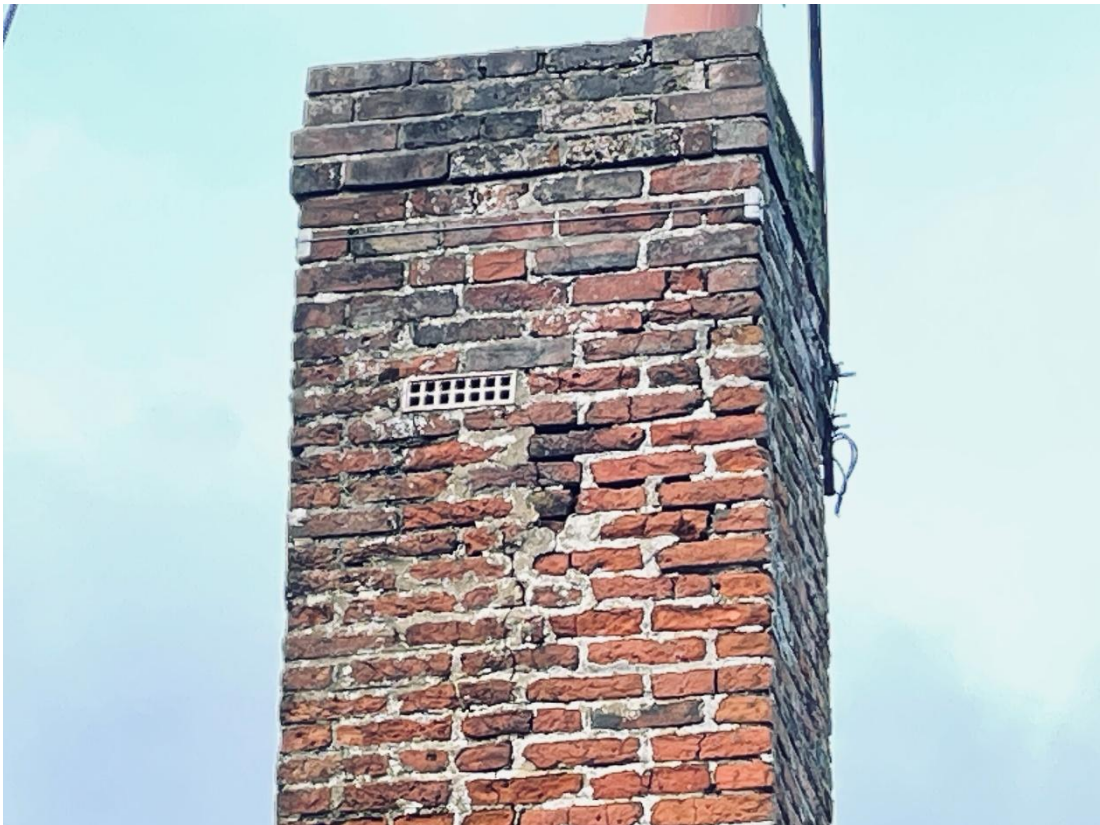
Poor pointing to the chimney.
