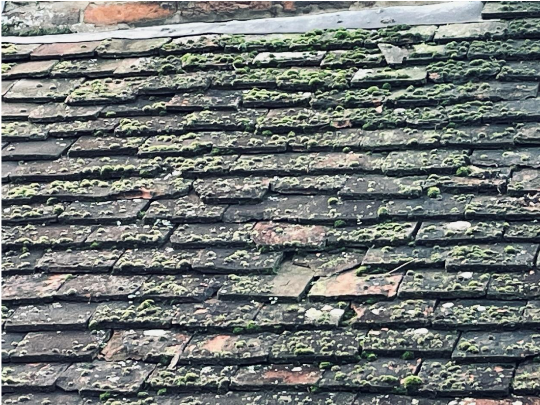
Broken tiles to the front slope of the roof.
